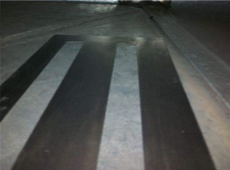
Figure B.2 Visual comparison examples the air duct cleanliness.
