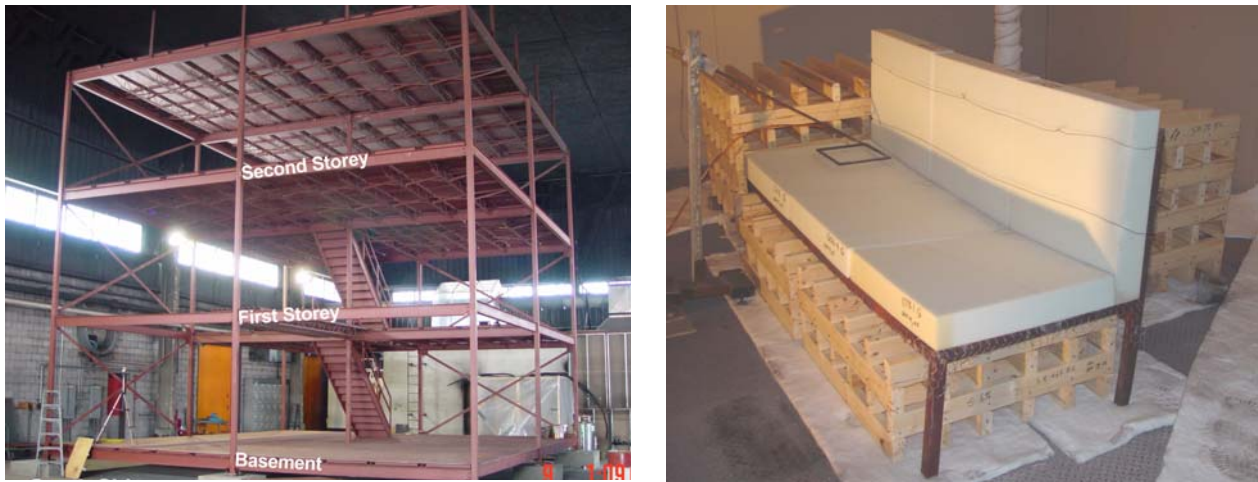
Figure 3. Test Facility under Construction and Fuel Package Mock-up Sofa
