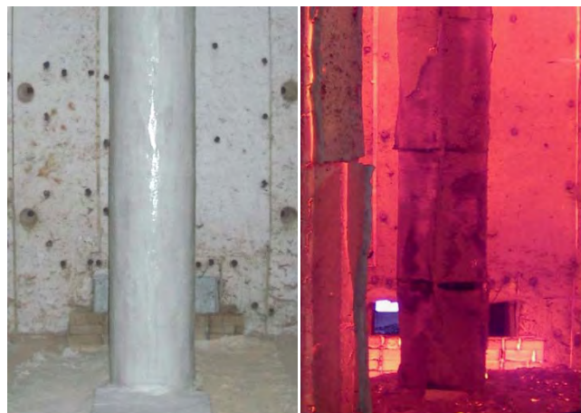
Figure 1: Typical circular column before and after fire testing
