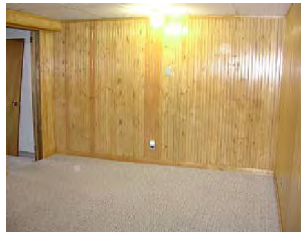
Figure 16. Combustible (wood) wall finish
