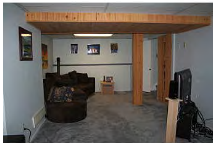
Figure 15. Combustible (wood) ceiling finish
