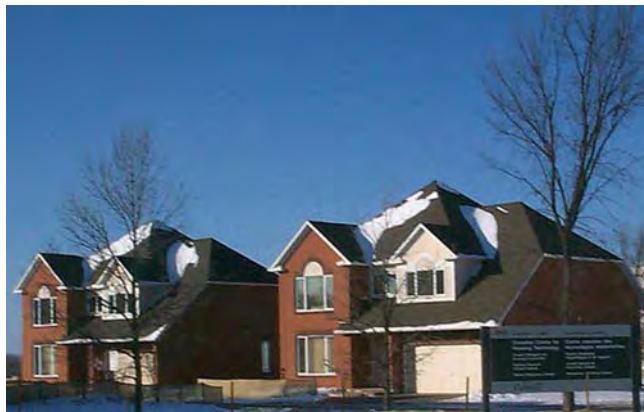
Figure 1 The research houses on the National Research Council of Canada campus
