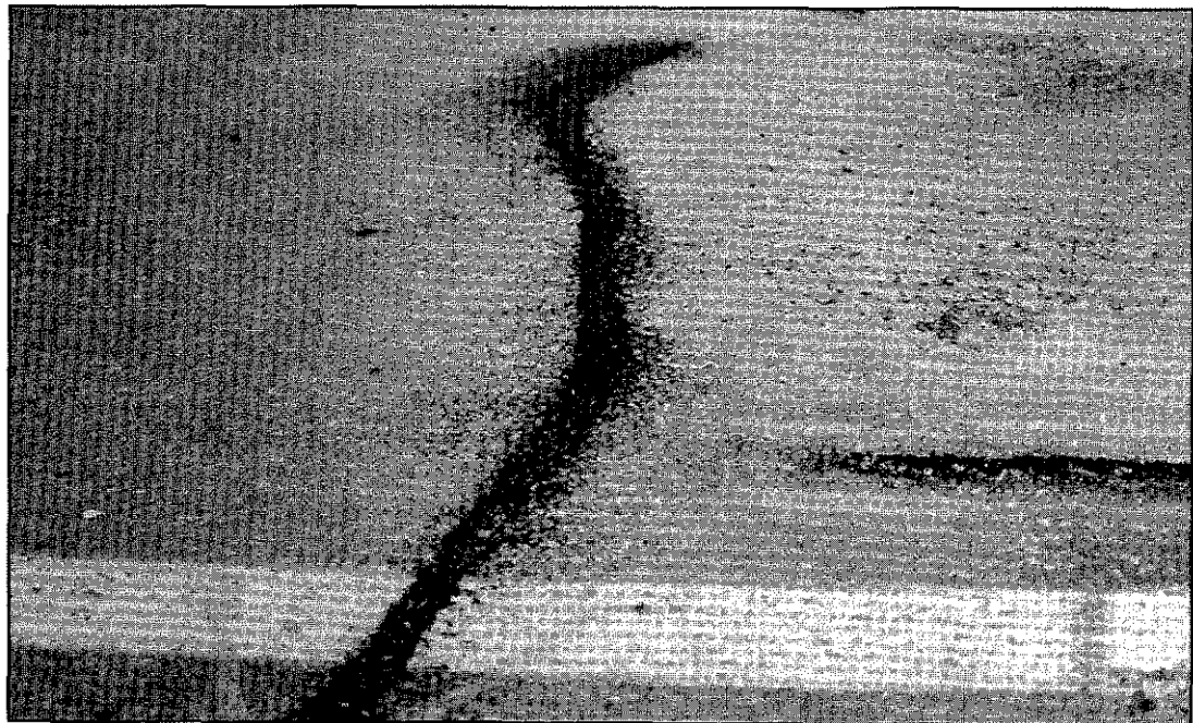
Figure 18. Typical blackening of an overheated rout
