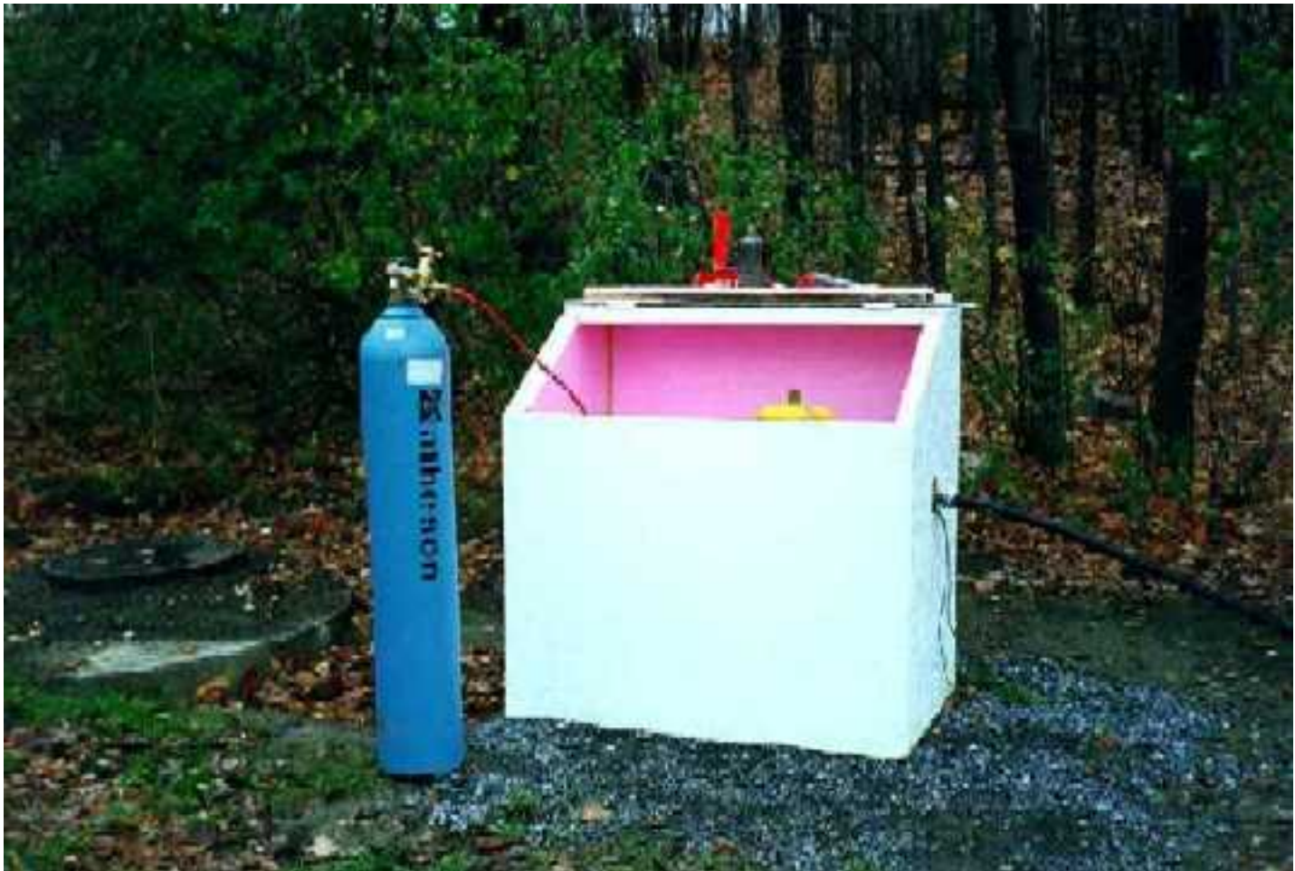
Hydrogen/nitrogen gas mixture introduced into "live" water pipe at fire hydrant.
