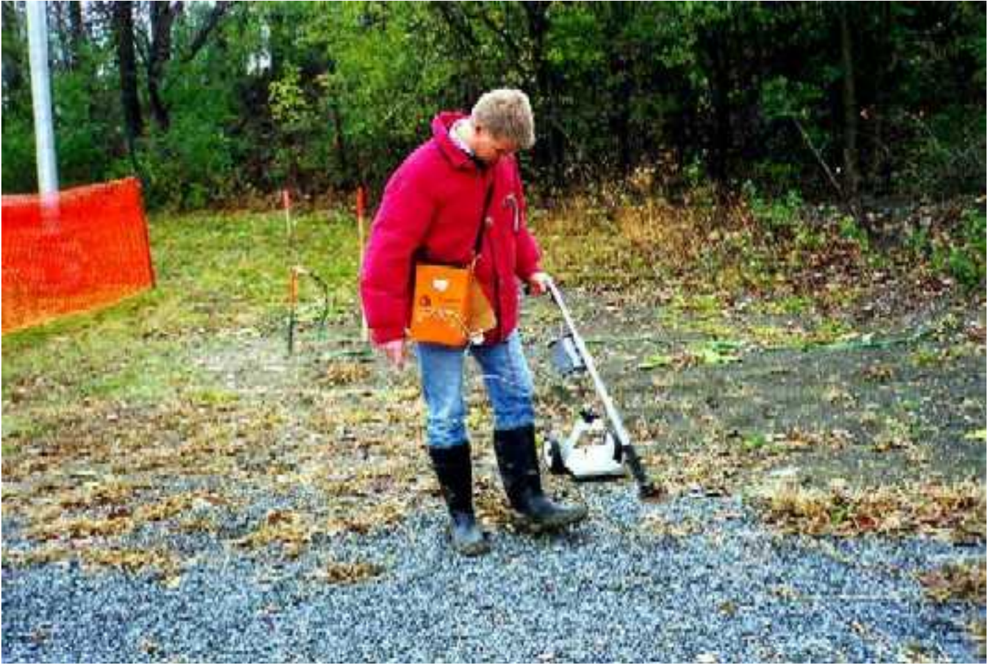
Hydrogen gas sensor being used to detect gas that might escape through pipe leaks.
