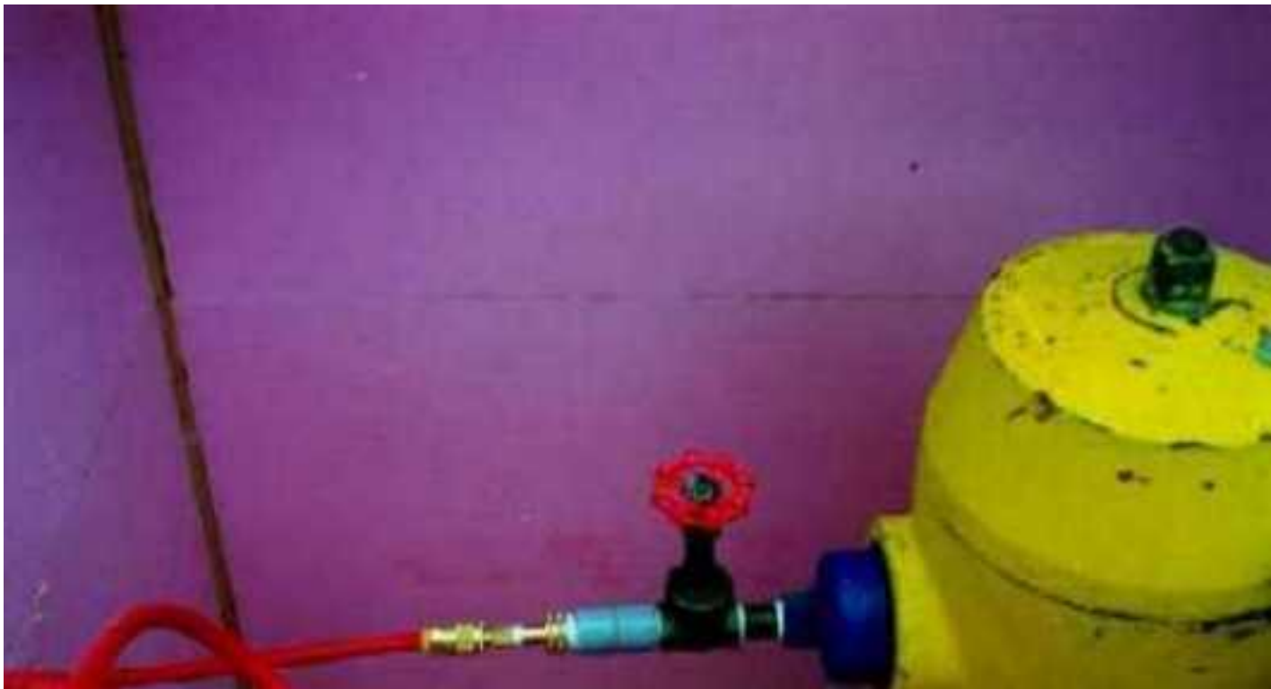
Special adapter used to inject gas mixture into fire hydrant.
