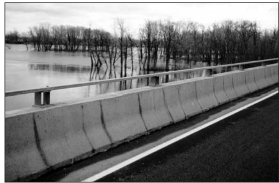
Figure 3. Typical span of barrier wall after reconstruction.
