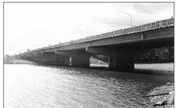
Figure 1. Vachon Bridge during rehabilitation in 1996, Laval, Québec
